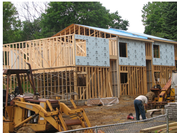
Figure 1. Wood framed construction
