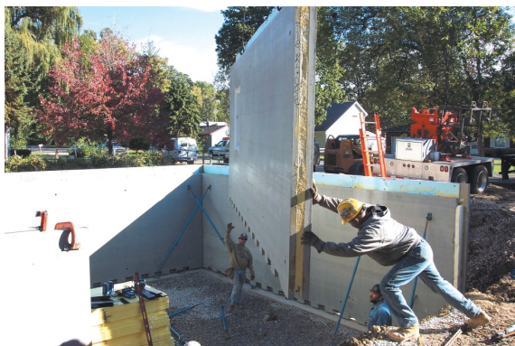
Figure 4. PCP construction (image courtesy of Dukane Precast)
