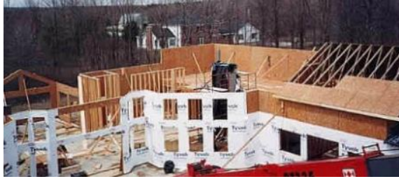
Figure 3. SIP construction (image courtesy of Thermocore Panel Systems)
