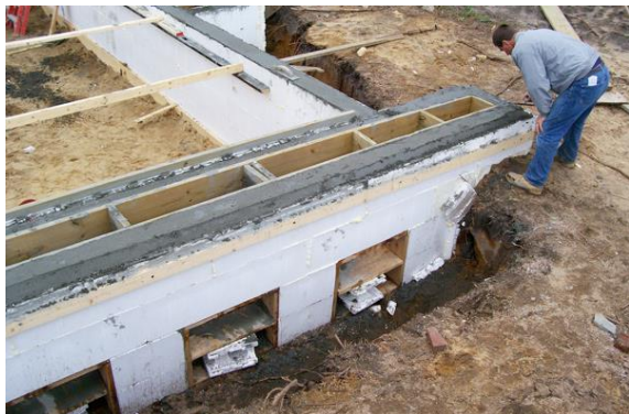
Figure 7. ICF construction (courtesy of LaBarge Cape Cod Engineering)
