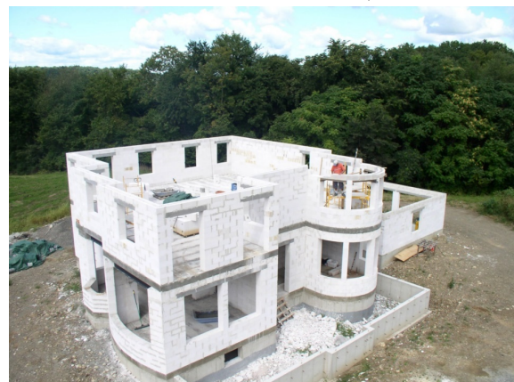
Figure 6. AAC construction (image courtesy of Portland Cement Association)
